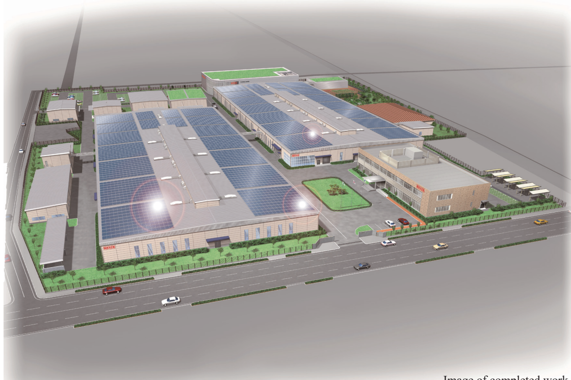
Image of completed work
